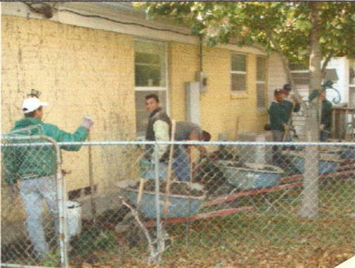
7 ea. Helical Piers with GH Brackets
